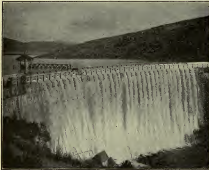
FIG. 286. — A masonry dam built by the United States government, forming a large lake in which water is stored for use in irrigation during the summer.
